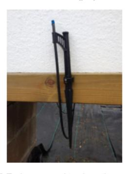
Figure 8 End were used to close the mainline after everything is connected; the system was ready for testing.
